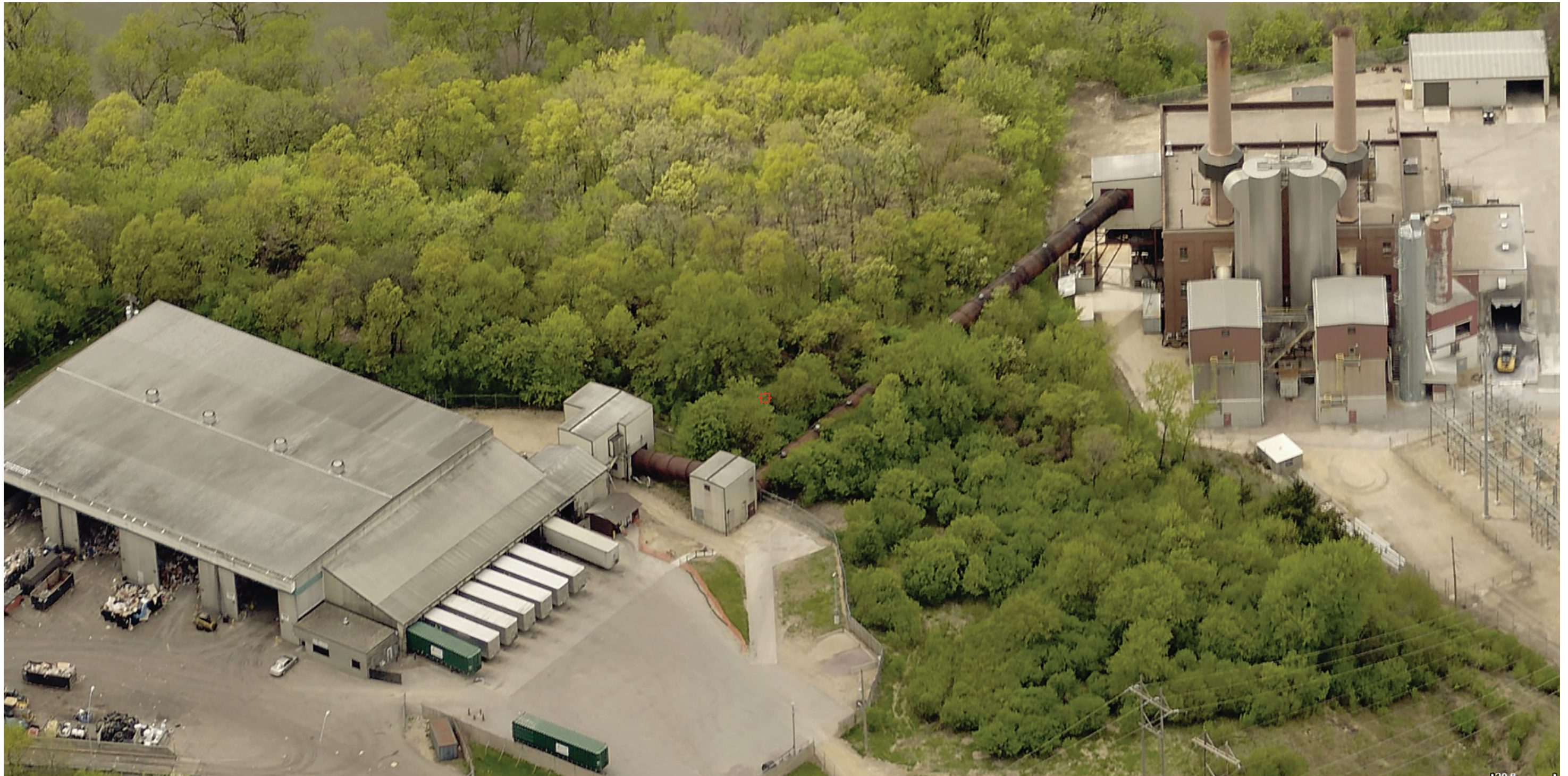
Xcel Energy's Wilmarth power plant burns trash. Sounds like a good idea, but not everyone agrees with the practice Courtesy Blue Earth County.
